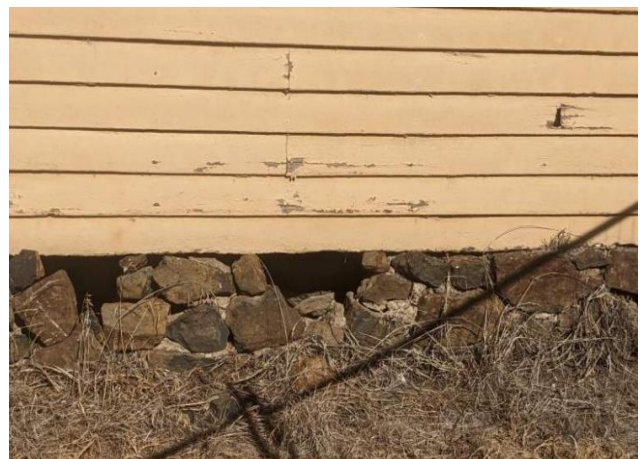
Figure 13 External view of the collapsed sub-floor wall
