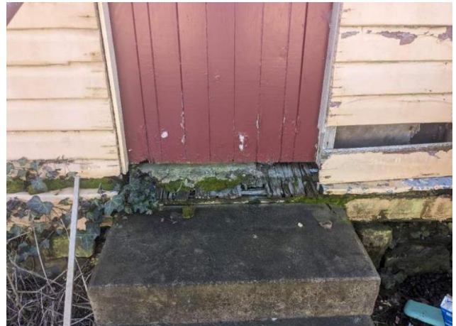
Figure 11 External view of the decayed floorboards and floor framing with detached weatherboards and decay wall framing at front annex.
