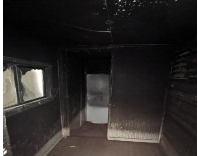
Figure 21 Internal view of smoke damaged finishes in west rear annex rooms
