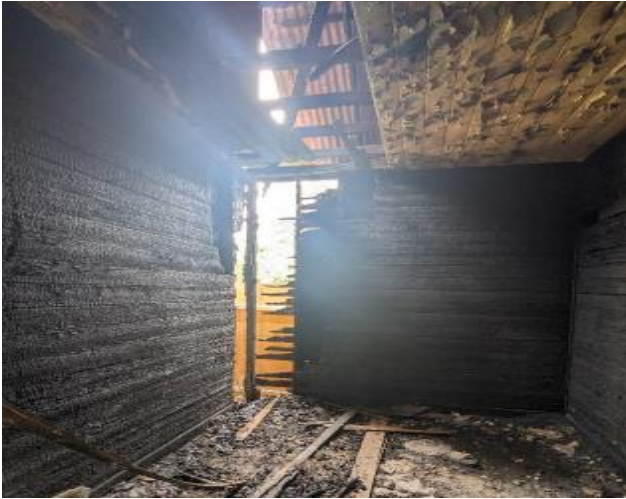
Figure 20 Internal view of charred wall finishes and in rear west bedroom
