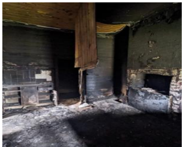
Figure 19 Internal view of the collapsed ceiling, charred surfaces in west central room
