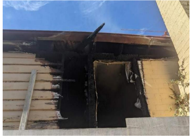
Figure 9 External view of charred ceiling, timber framing and weatherboards.
