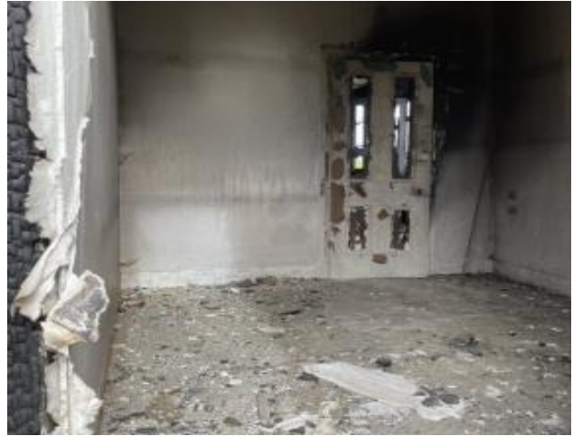
Figure 15 Internal view of the decaying timber doorframe and fire damage.
