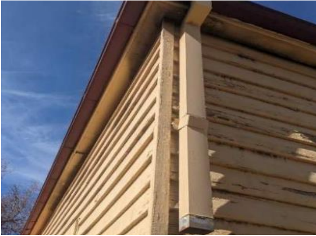
Figure 8 External view of peeling paint and minor decay of weatherboards, including the discontinuous downpipe.
