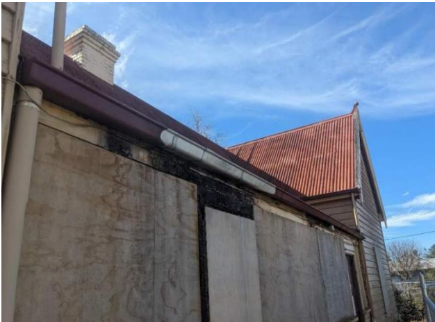
Figure 10 External view of charred door framing and weatherboards with damaged gutter at front annex.
