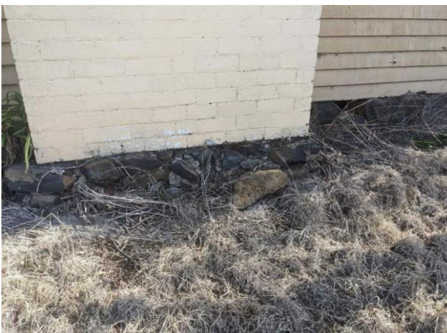
Figure 12 External view of rubble collapse beneath the brick fireplace
