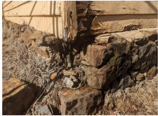
Figure 7 External view of the collapsed sub floor wal and decay of weatherboards and trim.
