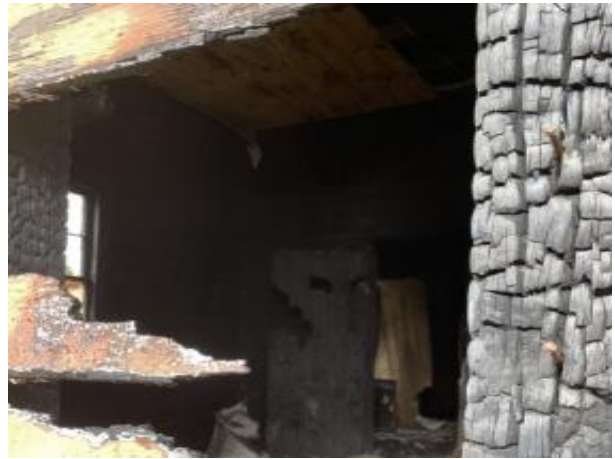
Figure 17 Internal view of the fire damage to the window.
