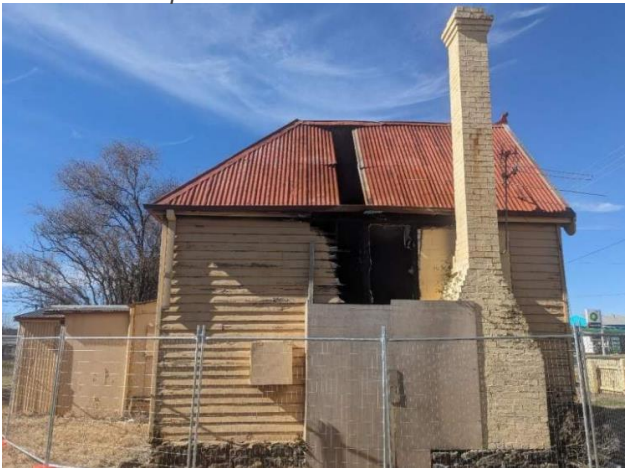
Figure 6 External view of the fire damaged roof and wall at the west end of the building
