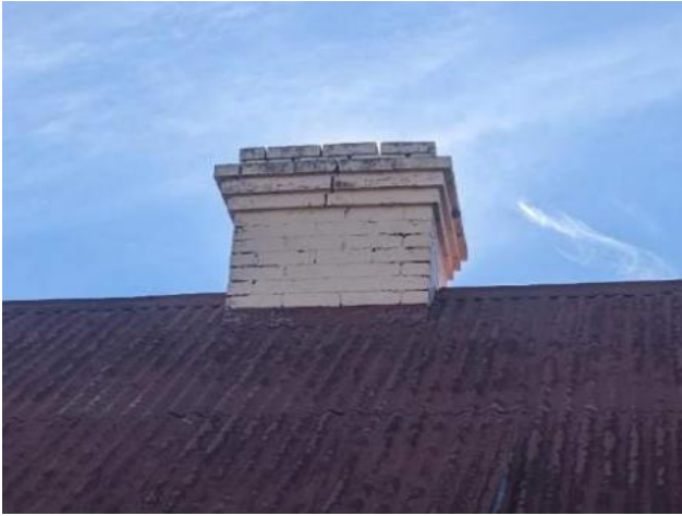
Figure 14 External view of mortar loss and cracking in the central chimney.
